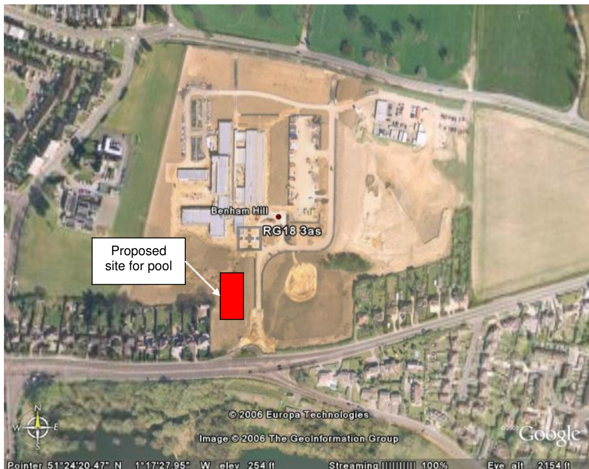
West Berkshire Community Hospital - when under construction (RG18 3AS)
